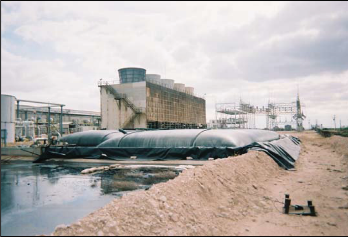
A geotextile tube used for dewatering and volume reduction of various types of sludge material
